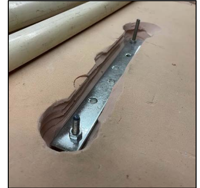
Figure 9. Steel plate and rods inserted.
